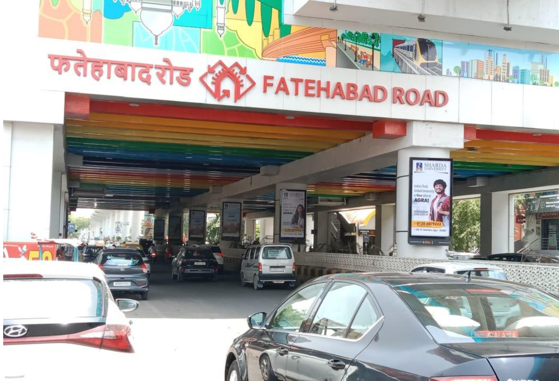
Fatehabad Road ( Metro Station )
