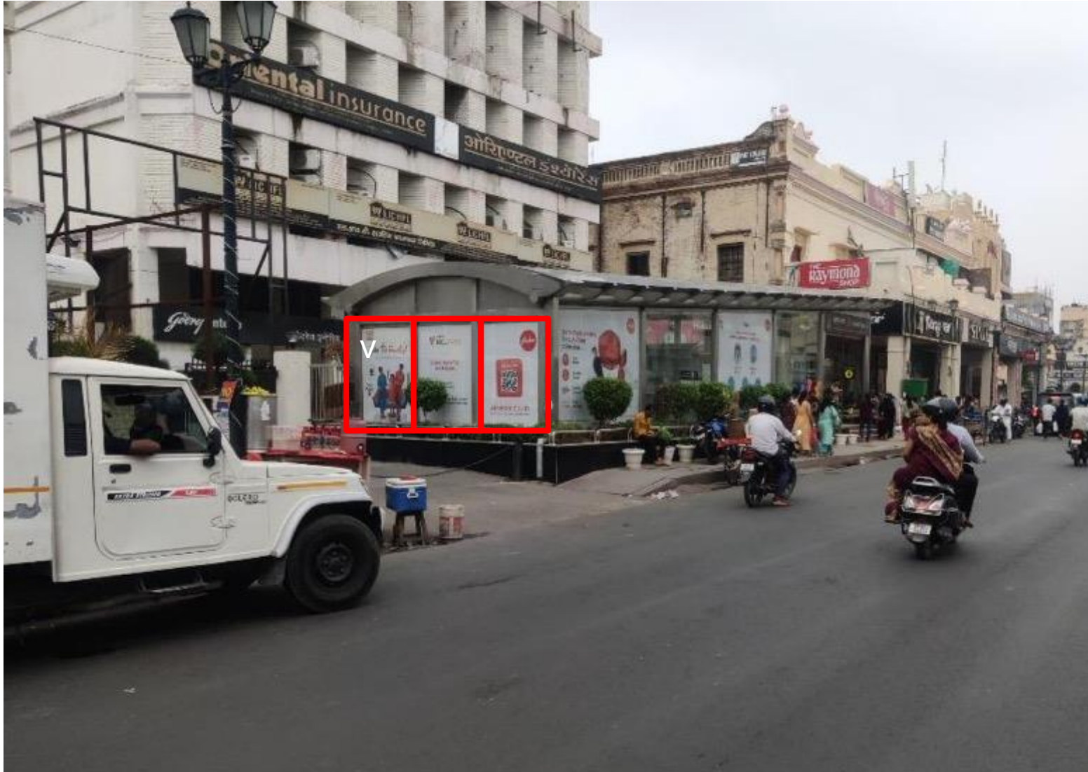
Hazratganj Metro Station – LIC HFL Entry – Back Side Glass of Entry – 5x8 - 3, Glass
