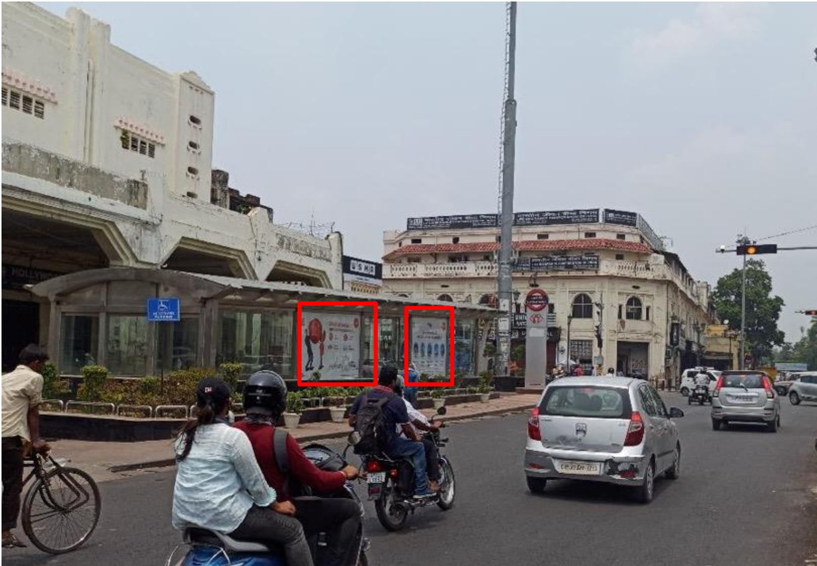
Hazratganj Metro Station – Mayfair Entry – Glass Parallel to Road – 12x7 & 12x8 - 1, Glass
